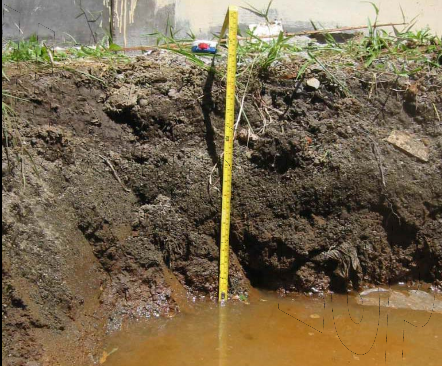
Typical Aceh situation– implementation with groundwater @ 45cm
