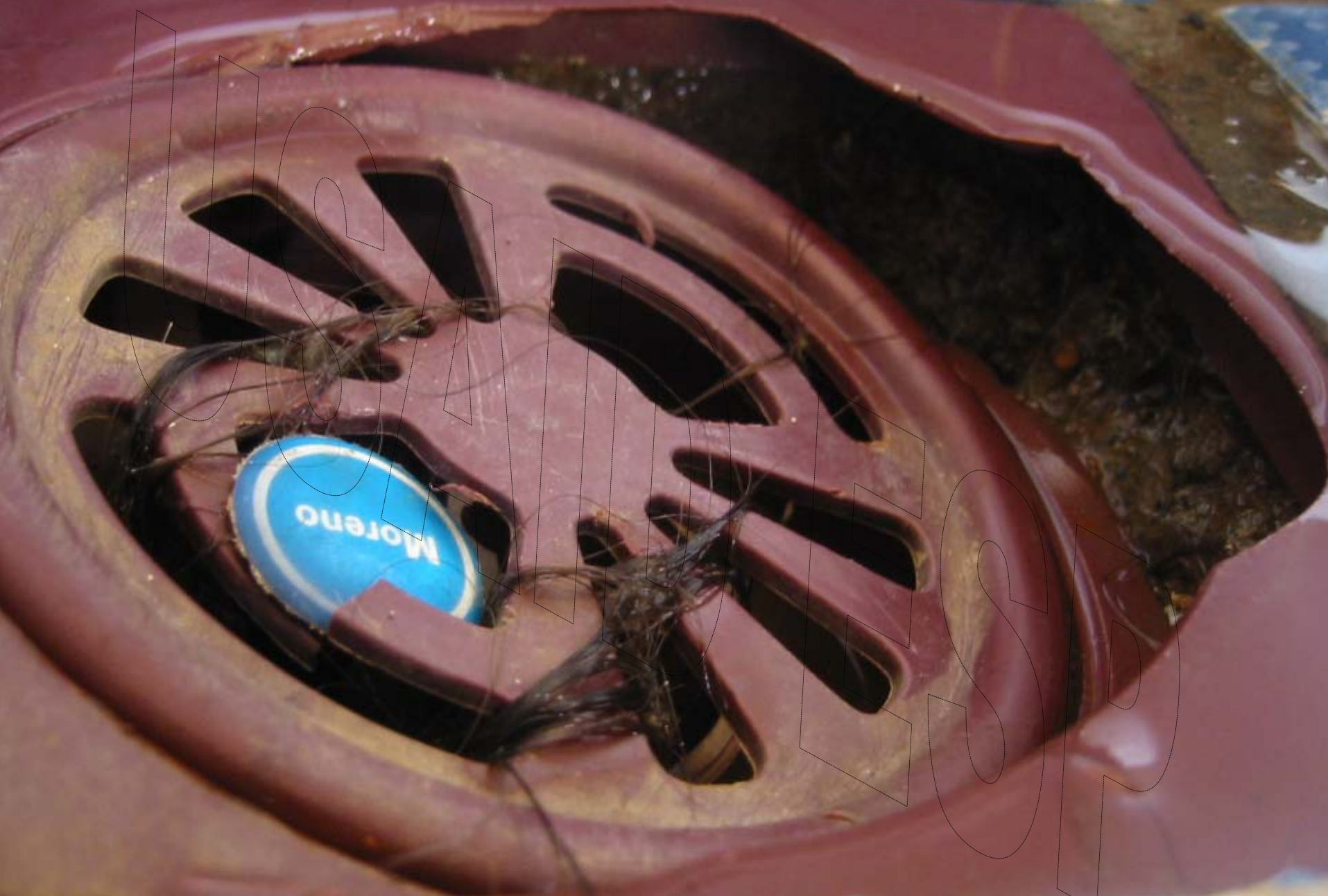
Why a grey-water (check-)filter is recommended
