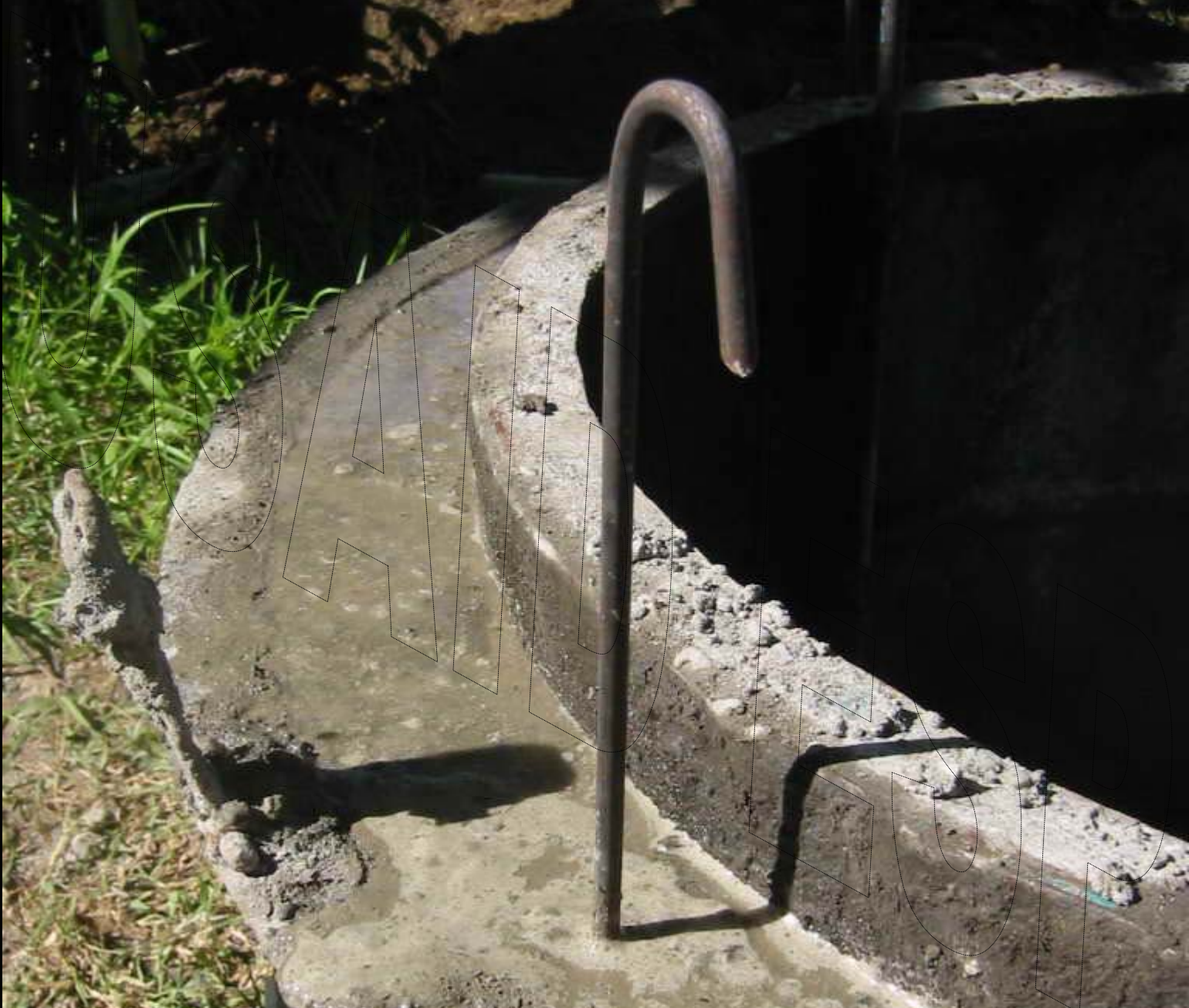
Hooks will be bent sideways to create rebar for AFR (see ESP design)
