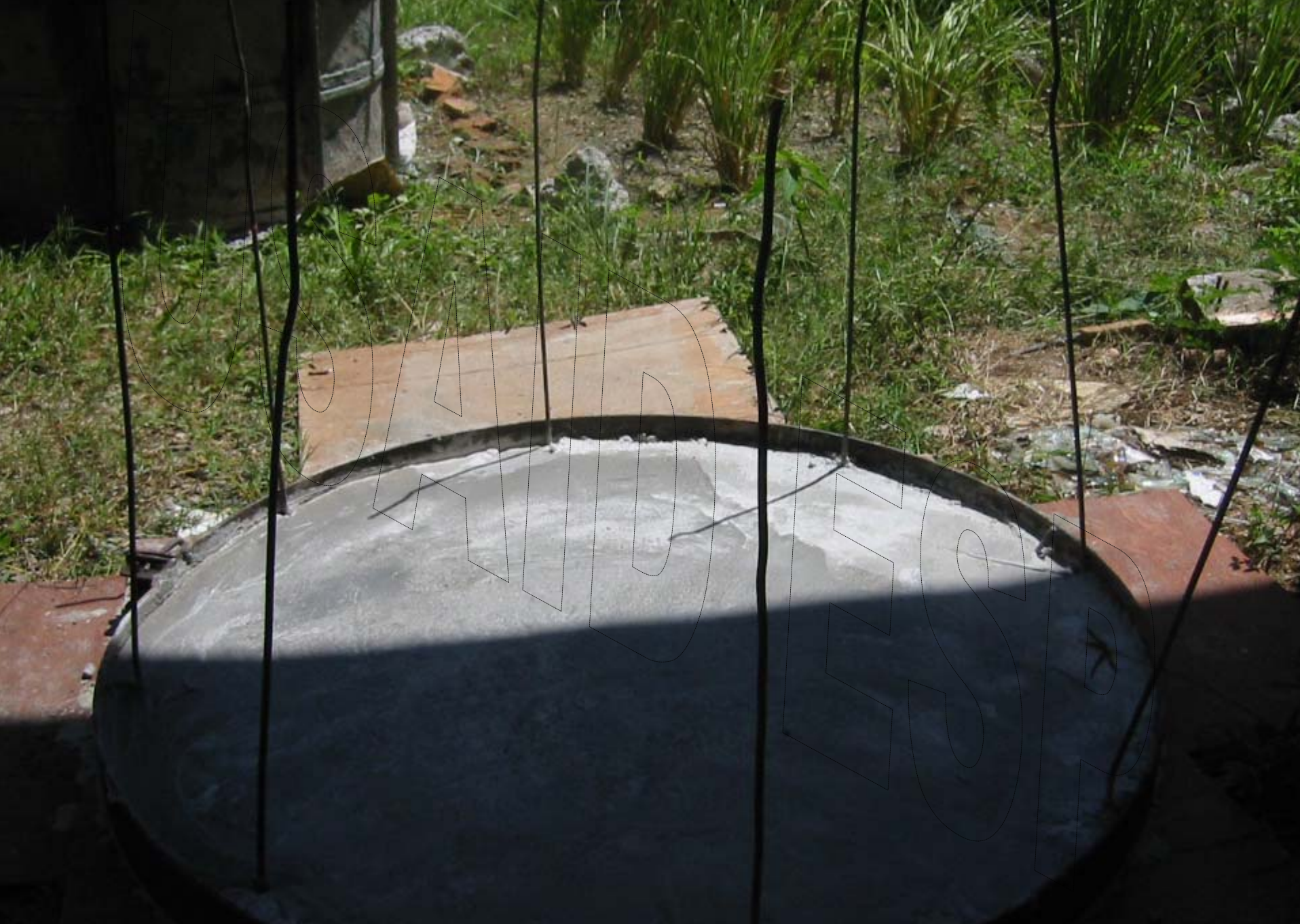
Reinforced bottom for concrete ring – rebar extends 70cm up
